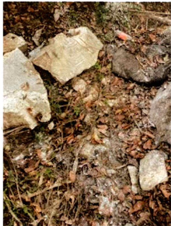
Manhole 1749 After Cleanup
