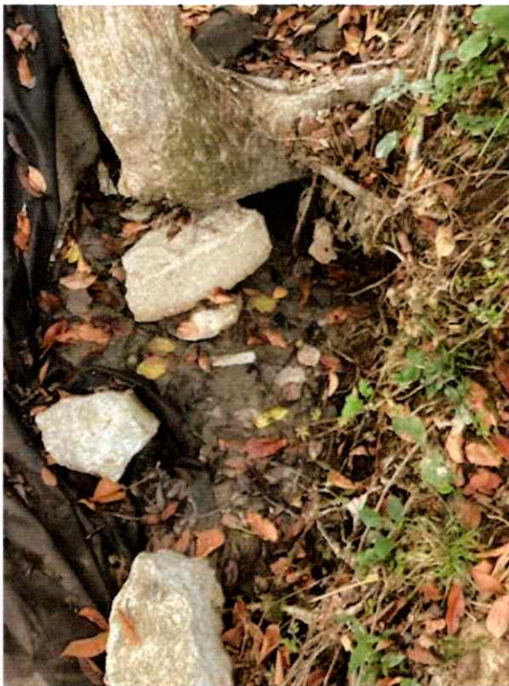
Manhole 1749 Before Cleanup
