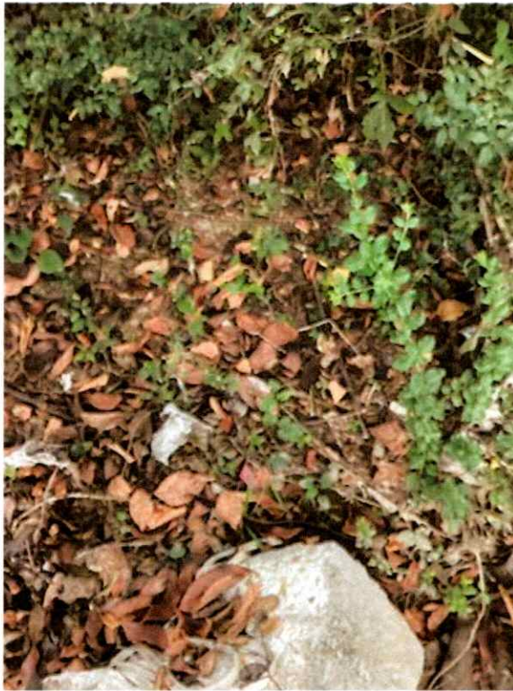
Manhole 1749 Before Cleanup
