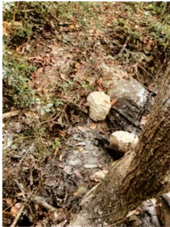
Manhole 1749 After Cleanup
