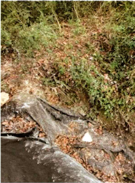
Manhole 1749 After Cleanup
